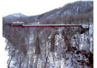
the Tanzan River, a tributary of the Ashibetsu River, was constructed in 1944 in response to a request to increase coal production. It was part of the Mitsui Mining . Company's private railway. Completed in December 1945, the bridge is 94 meters long and 30 meters high. A diesel locomotive and coal freight cars are displayed on the iron bridge. It is a Registered Tangible Cultural Property of
