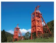
Built in 1923, this is the second oldest mine shaft in Hokkaido. The two ventilation shafts, one for intake and the other for exhaust, were in use until the mine closed in 1972. The switchyard and raw coal pocket (where the freshly mined coal was initially stored) were built in 1925. It is now open to the public as the Coal Mine Memorial Forest Park
